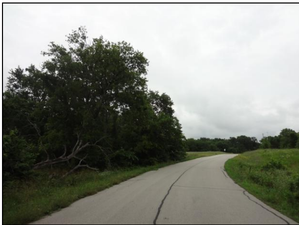
Viewing east along James M Pitts Road.
