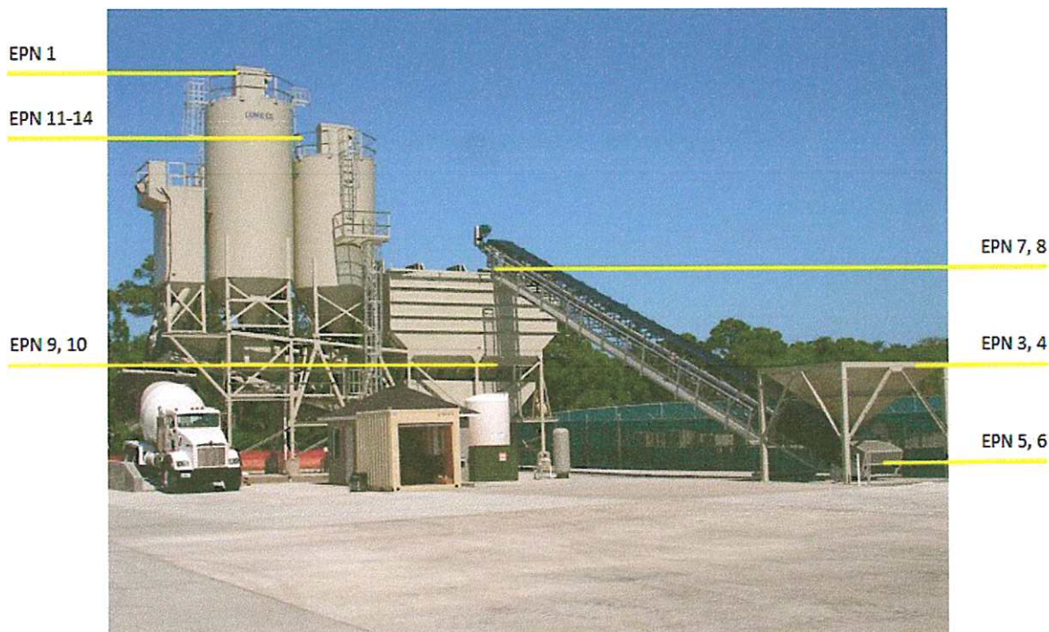
Figure 1. Depiction of a Typical Concrete Batch Plant And Modeled Emission Source Release Heights
