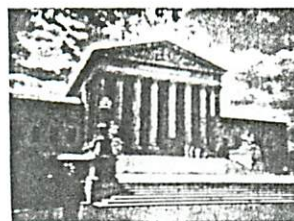
Supreme Court Bldg. Washington D.C. Plaza Waterproofing
