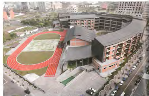
The Dongxing Elementary School buildings feature a high-tech impression, elements of traditional Hakka style and a vision of community sharing.
