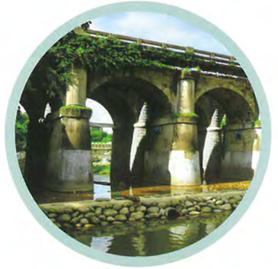
Old Dongan Bridge, Guanxi Township
