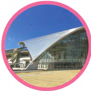
Taiwan High Speed Rail Hsinchu Station, Zhubei City
