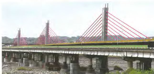
The cable-stayed Zhulin Bridge will be a new landmark by the Touqian riverside once it is completed.
