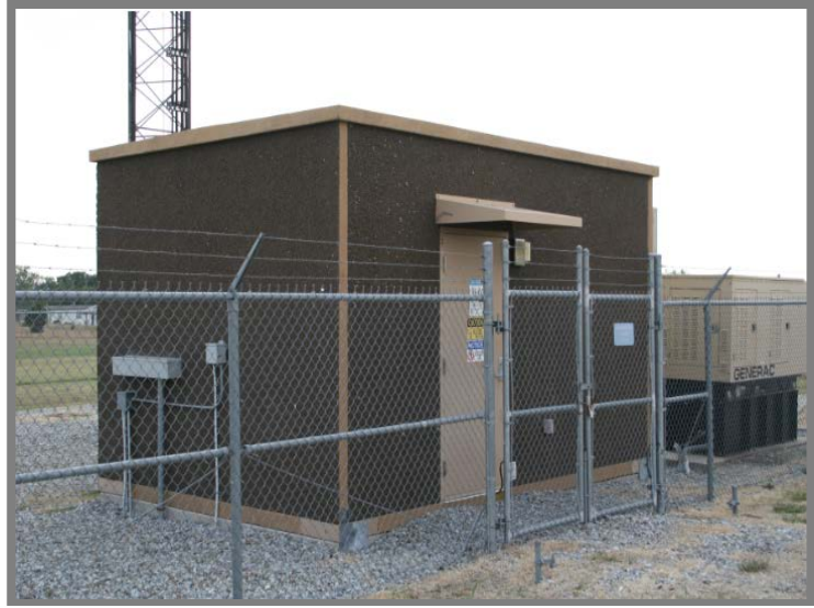
Verona Radio Site Equipment Shelter
