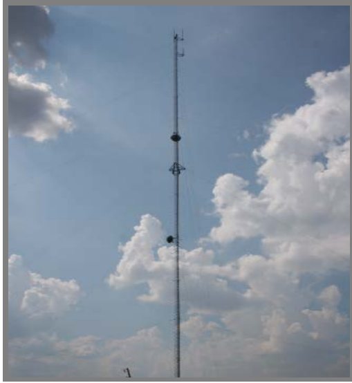
Verona Guyed Radio Tower
