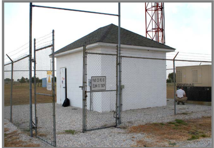
Celina Radio Equipment Shelter
