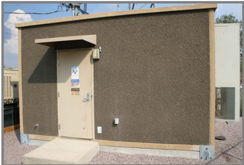
Copeville Radio Equipment Shelter
