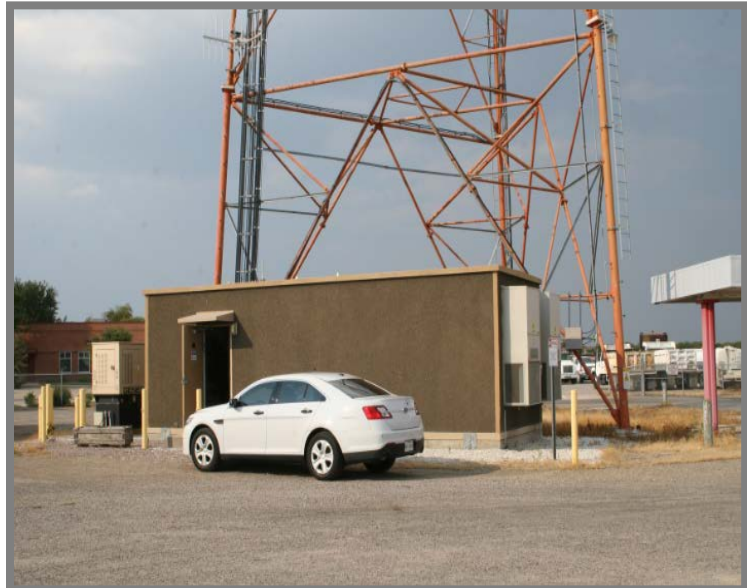
Wilmeth Road Equipment Shelter
