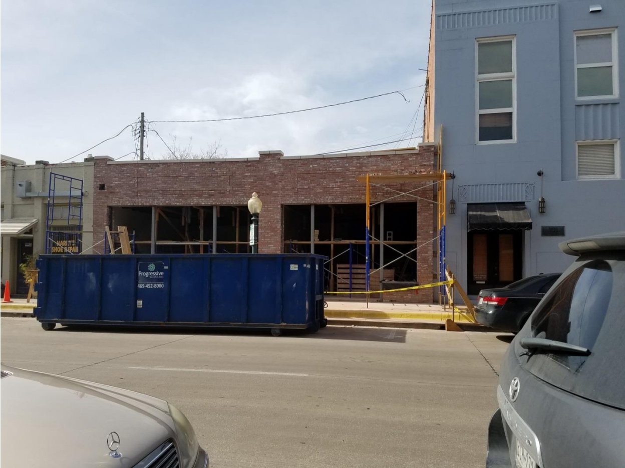
Goodner Building 106 S. Tennessee
