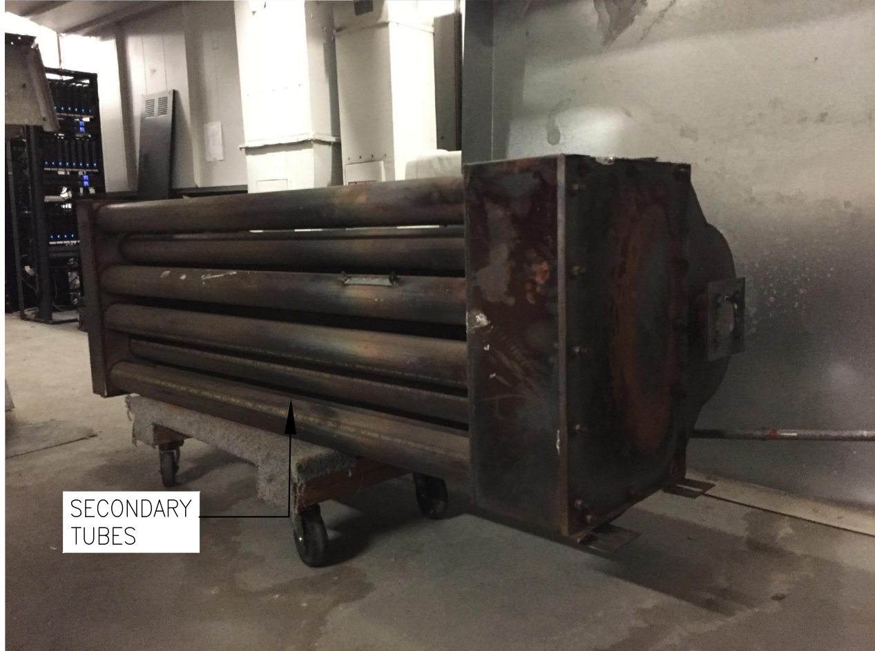
03 AHU-1 HEAT EXCHANGER
