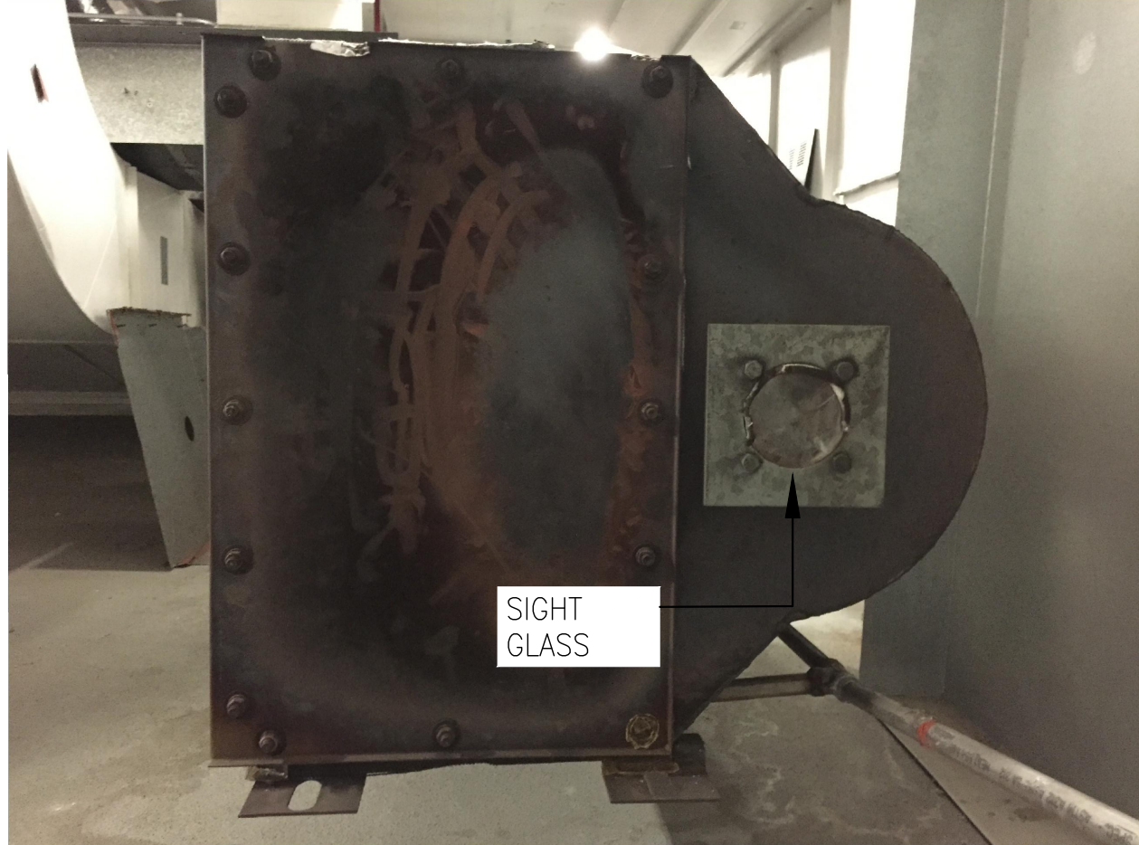
02 AHU-1 HEAT EXCHANGER BACK VIEW
