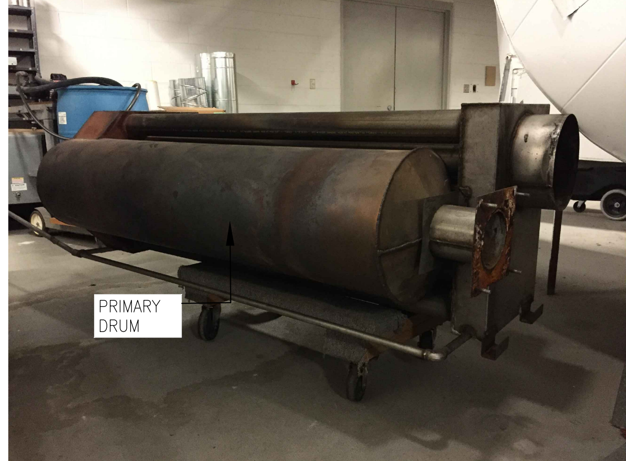
04 AHU-1 HEAT EXCHANGER
