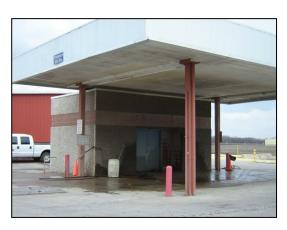
The County has a covered wash bay at the Public Works Service Center which utilizes a pre-wash and wash water is treated through a grit trap. Proper maintenance of the grit trap is conducted on a regular basis. The County inspects the grit trap at least 10 times per year and maintains the trap as needed, but at least once per permit term.
