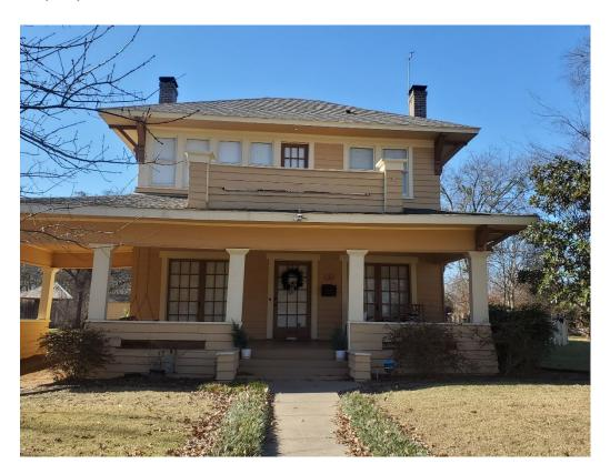
Following an appeal by the owner, another inspection was conducted in January of 2022. It was determined that the missing board of the balcony wall is actually part of the construction of the house and is needed for draining the balcony.
