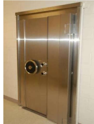
The Level 5 door of the Long-Term Storage Vault (same model used for each vault).
