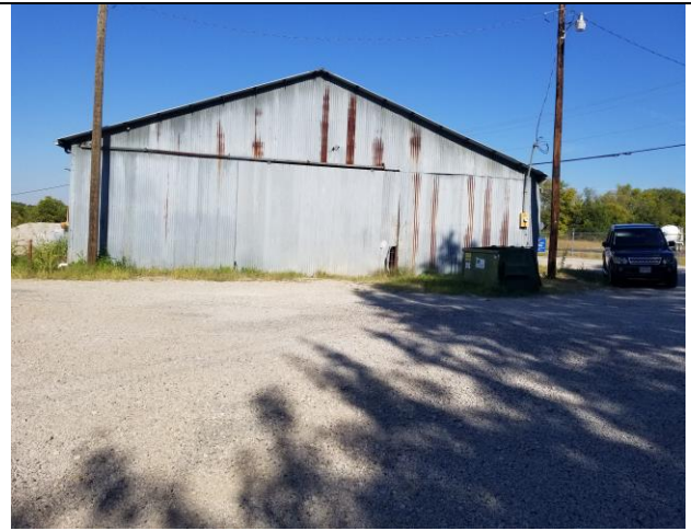
SE elevation of metal building
