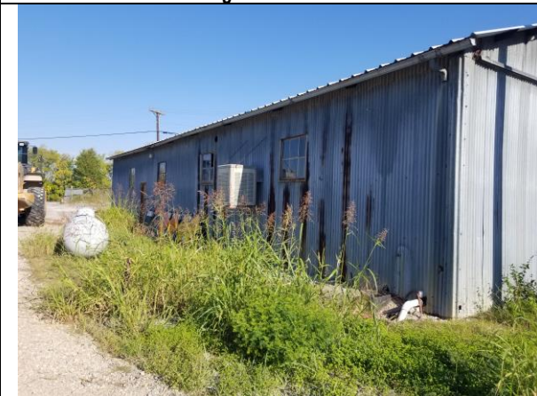
SW elevation of metal building
