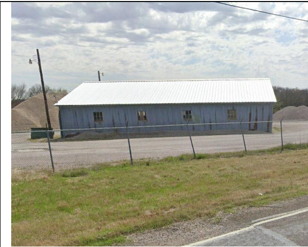
Metal building from road – NE elevation
