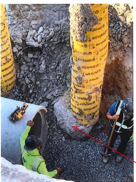
Photograph 5 - Excess Concrete Below Sonotube
