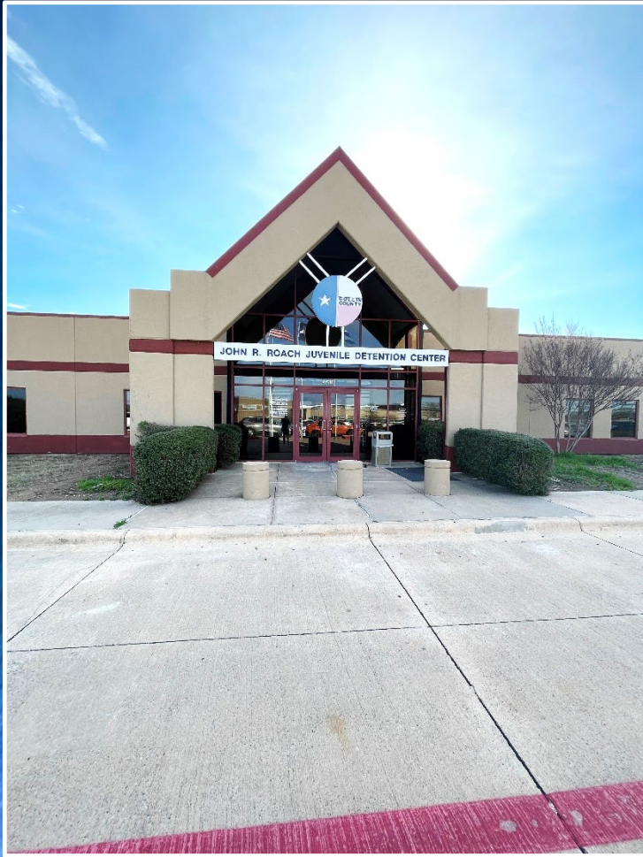
Facility Main Entrance
