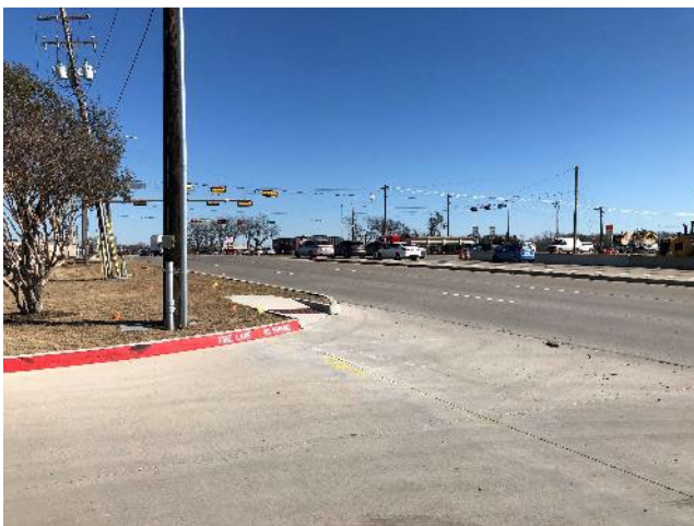
Looking east along State Highway 78
