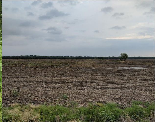
#8 Project at FM 2478
