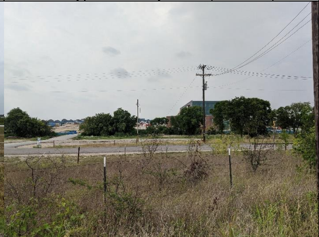
#4 New Construction south of Hackberry Cir.
