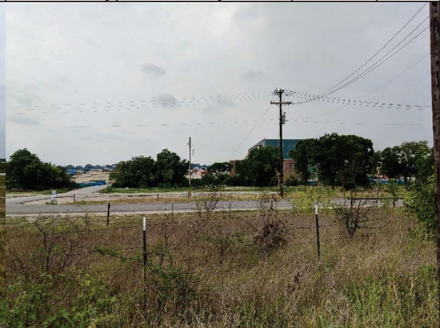
#4 New Construction south of Hackberry Cir.
