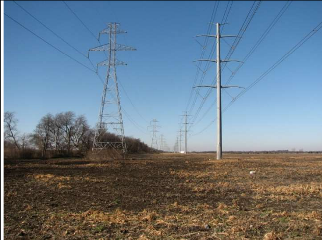
#7 Oncor electrical transmission line adjacent to the study area
