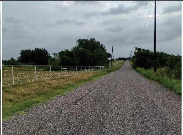
#2 Typical County Road (CR 1224)
