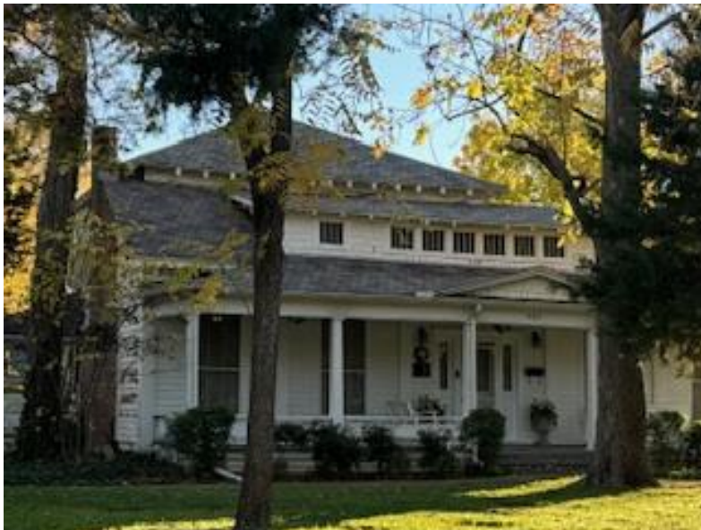
Howell House 909 Howell Street McKinney Peeling Paint
