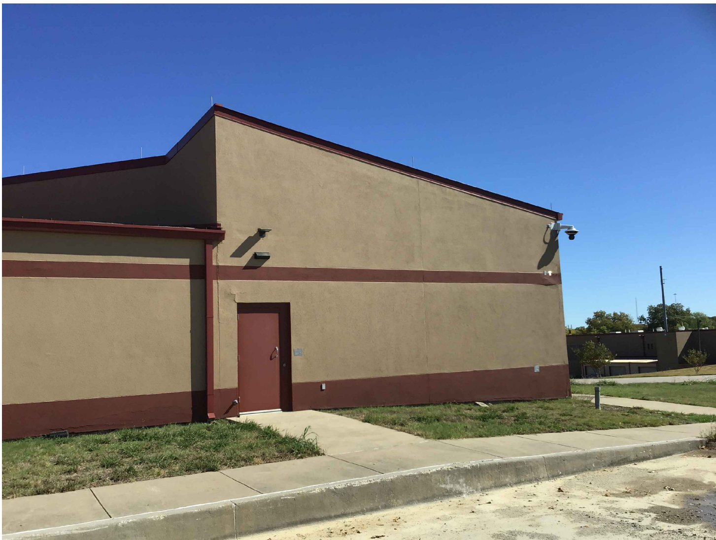
PARTIAL VIEW OF WEST FACADE
