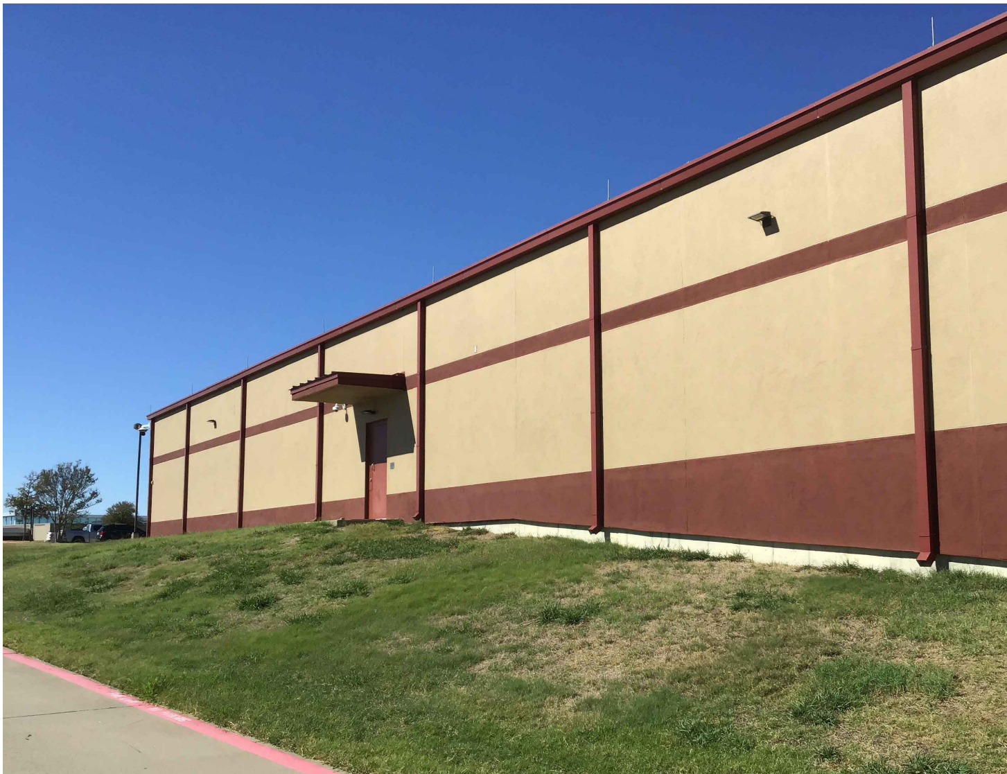
PARTIAL VIEW OF SOUTH FACADE
