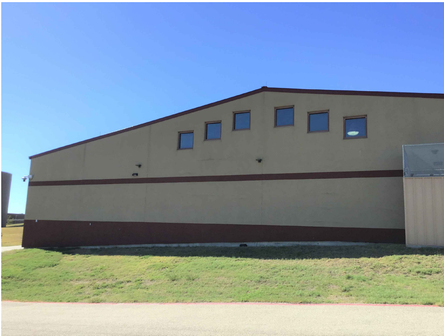
PARTIAL VIEW OF EAST FACADE
